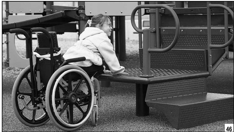
A transfer system typically consists of a transfer platform, transfer steps, and transfer supports.
