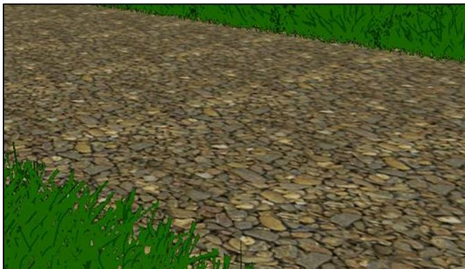
*Most loose materials, including gravel will not meet these requirements unless properly treated to provide sufficient surface integrity and resilience. Binders, consolidants, compaction, and grid forms may enable some of these materials to perform satisfactorily but require repeated maintenance.*
