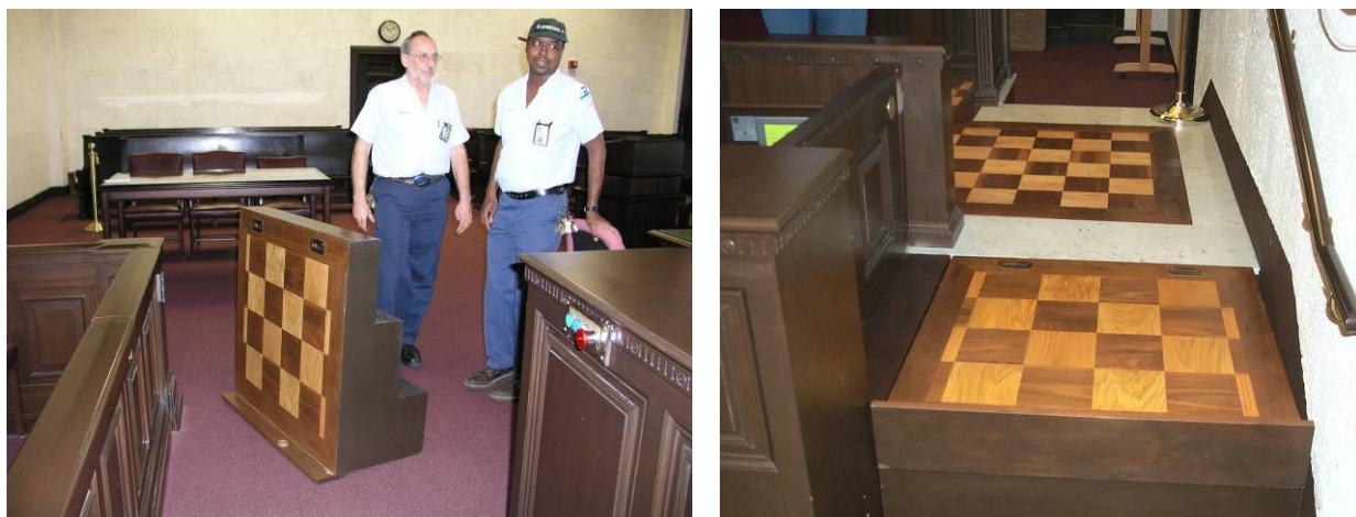
Figures: Common Error - The lift in the above courtroom requires the addition of a platform covering the stairs to be operable.
