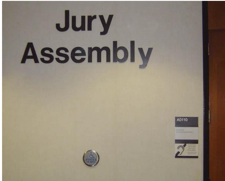
Figure: Jury Assembly room with power opening door and signage indicating availability of assistive listening systems
