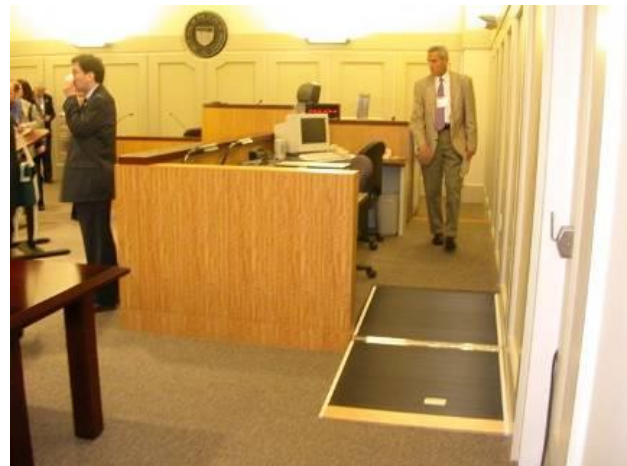
Figures: Common Error -These flip down ramps require assistance to create the accessible route, and when open, block the gate and maneuvering space for the door.
