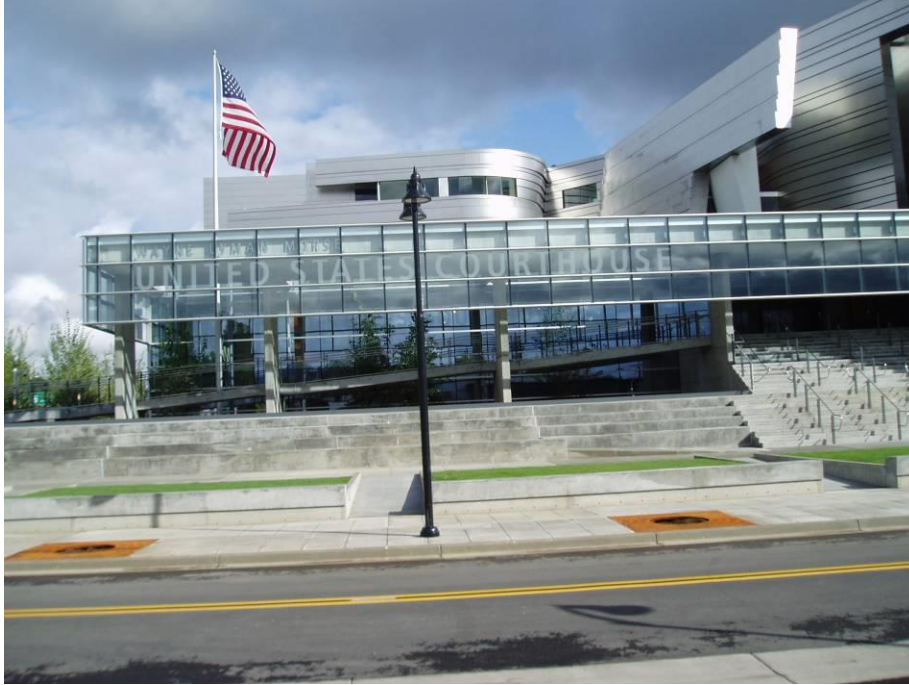
Figure: Plinth necessitates a ramp that is long and arduous
