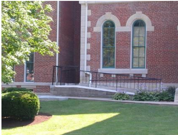
Figure: Common Error- This exterior ramp is located so that it provides access to a back door that is not visible from the outside.
