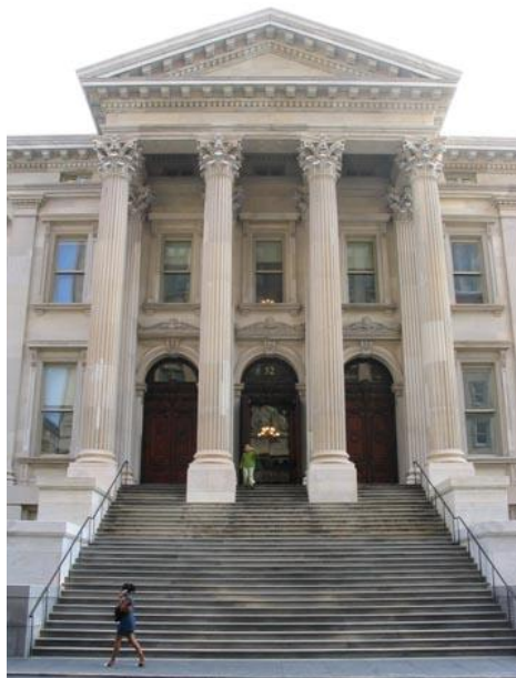
Figure: Plinth with stairs creating access problems
