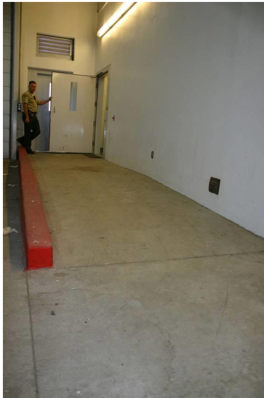
Figure: Detainee entrance with ramp.
