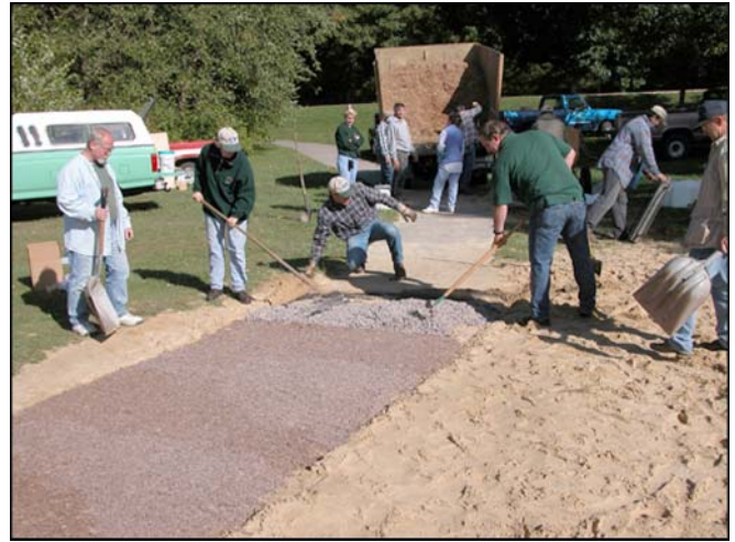
Figure 4—Leveling and compaction of binder-EWF mixture near junction with asphalt path.
