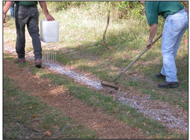
Figure 9—Application of Soil-Sement to bridle trail by drip-bucket method. Rakes were used to mix binder with EWF and level the trail.
