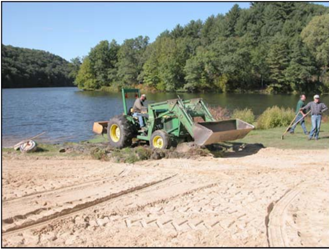
Figure 2—Grading of beach path to waterline.
